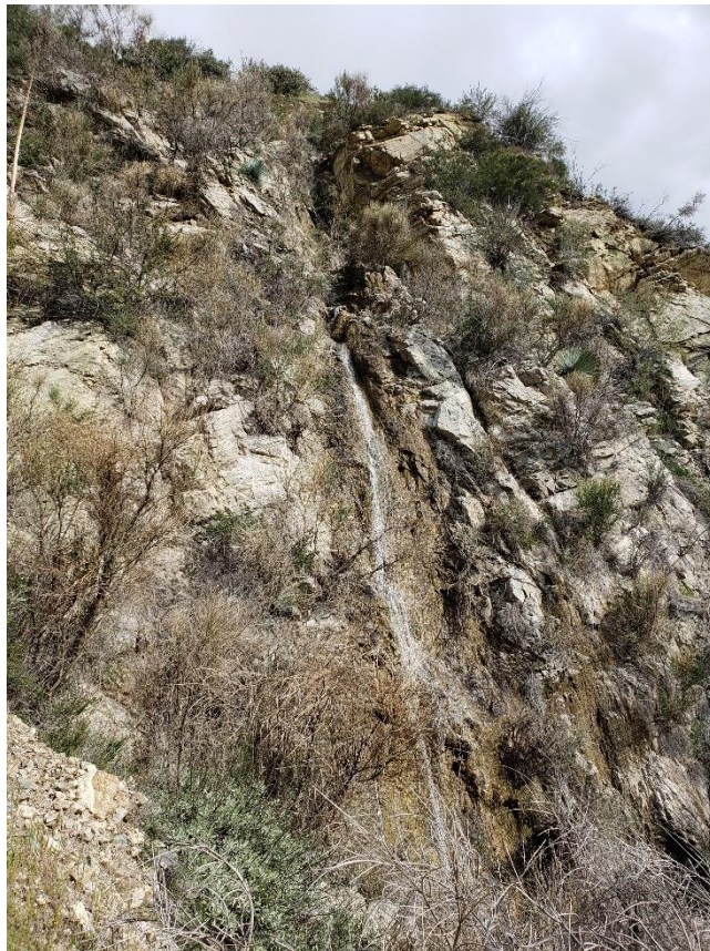
Figure 37: Potential mini wedge with small waterfall above the Sierra Powerhouse Access Road.
