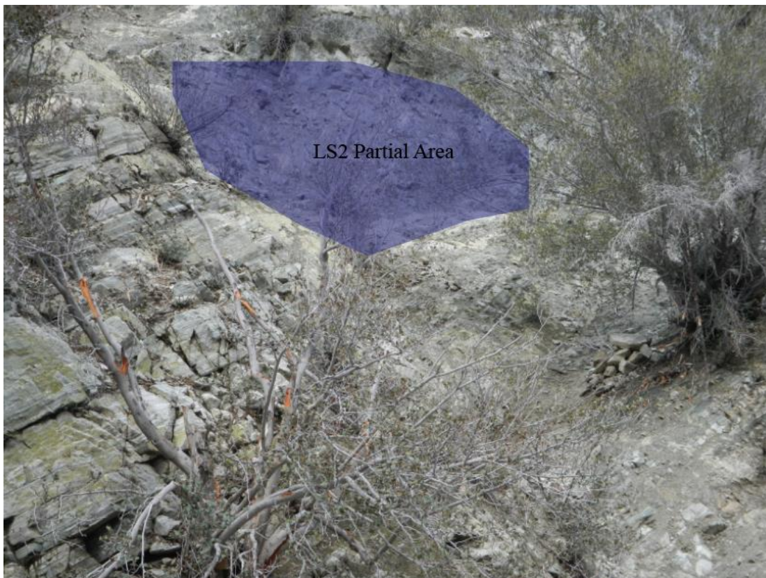
Figure 68: Photo of the failure surface taken by Dr. Nourse in 2017.
