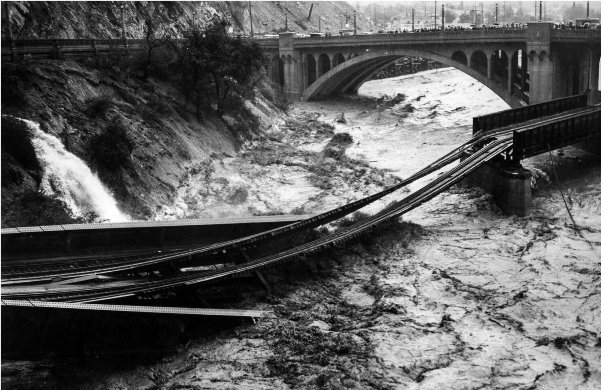
Figure 128: Floodwaters raging down the Los Angeles River on March 2, 1938, taken from North Figueroa Street bridge. (Los Angeles Times)
