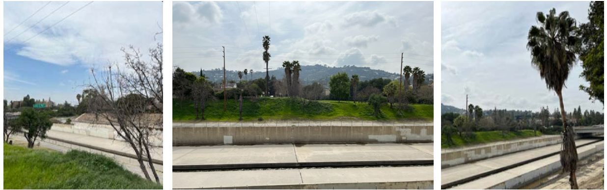
Figure 95: Site images showing current river conditions.
