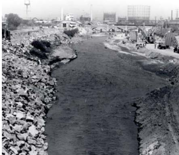
Figure 19: Results of the 1938 Flood (scouring, infrastructure collapse, channel breaches and widening).
