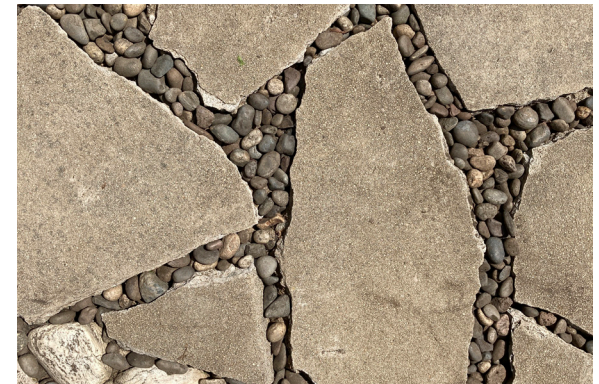
Figure 65: An example of porous paving: urbanite and gravel.
