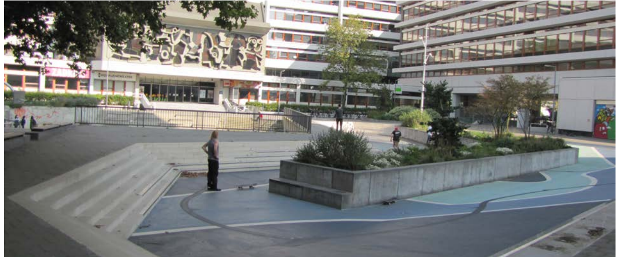
Figure 54: Benthemplein Water Square, Rotterdam.
