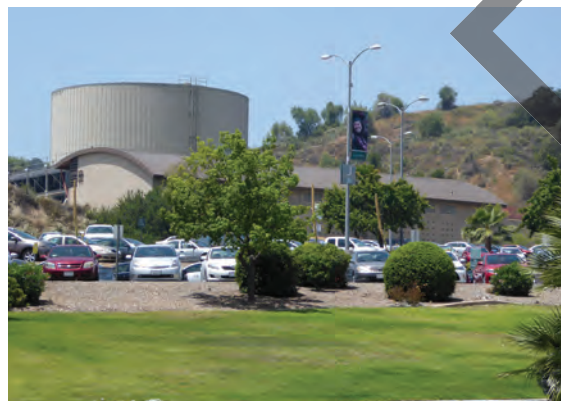
Campus core is served by a new chilled water central plant with thermal energy storage saving money and energy.
