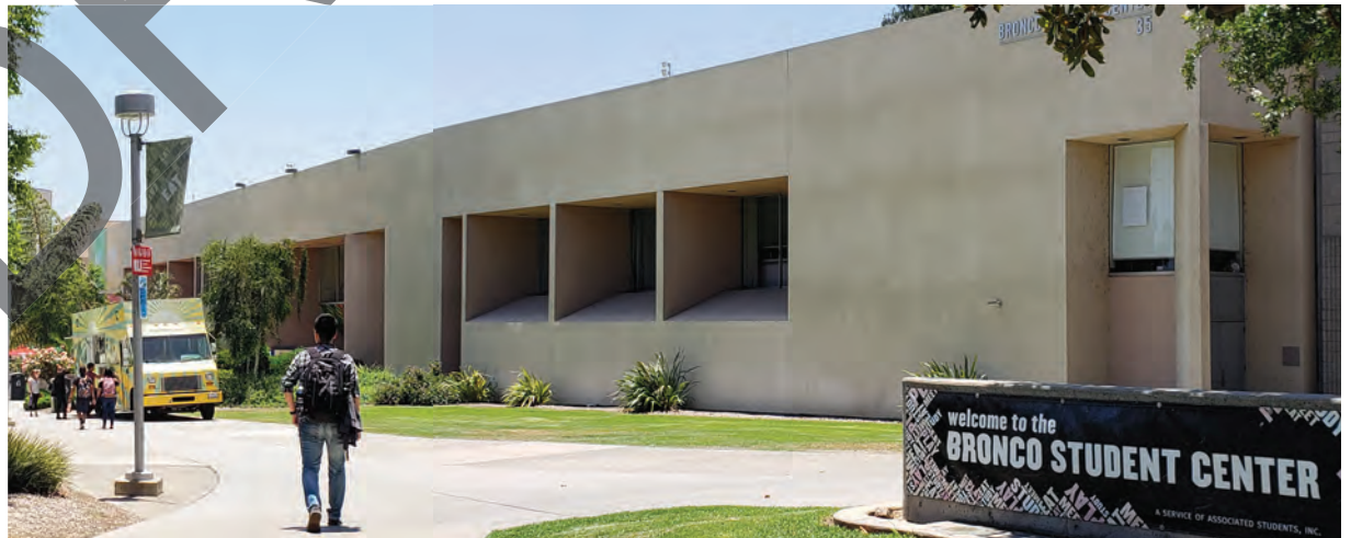
Proposed location of the Terrace Addition to expand the BSC while enhancing integration with the mall and University Park.
