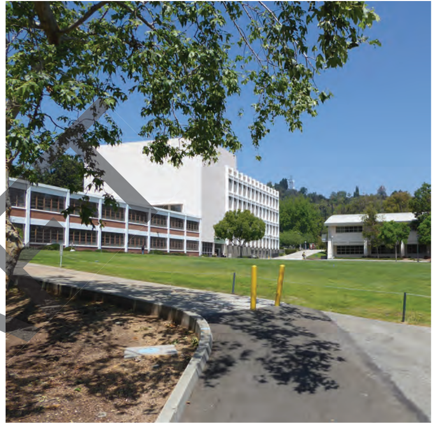
College of Engineering has more classrooms and teaching labs than any other building on campus.
