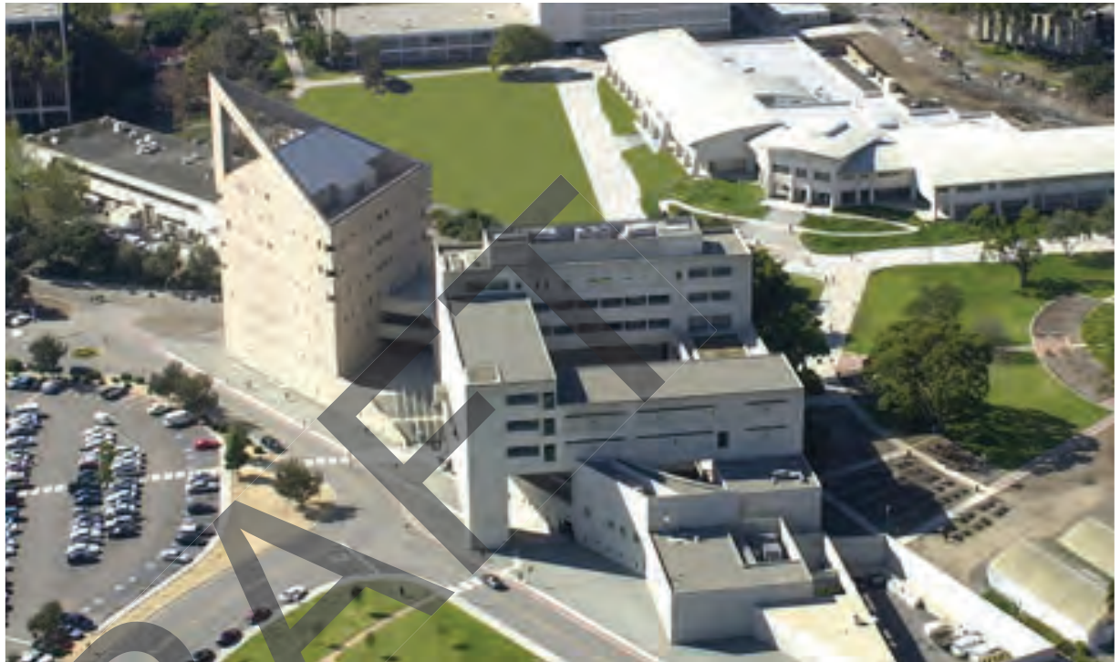
Bldg 98 was comprised of three structures (from left to right): the Tower and Registration building, Classroom building, basement (shared by all the structures) and the Podium. The Tower and Registration buildings have been demolished and the rest will be renovated.
