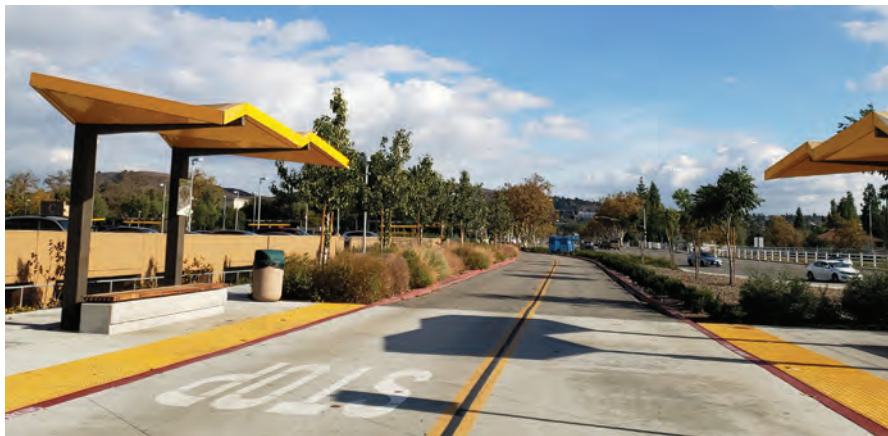
The HUB pilot would provide the basics with shelter-shades, FT bus pull-ins and a CPP shuttle stop until the full Mobility Hub is completed.
