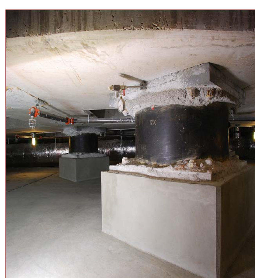
Figure 1: Base Isolation System-Ohio State Capitol
