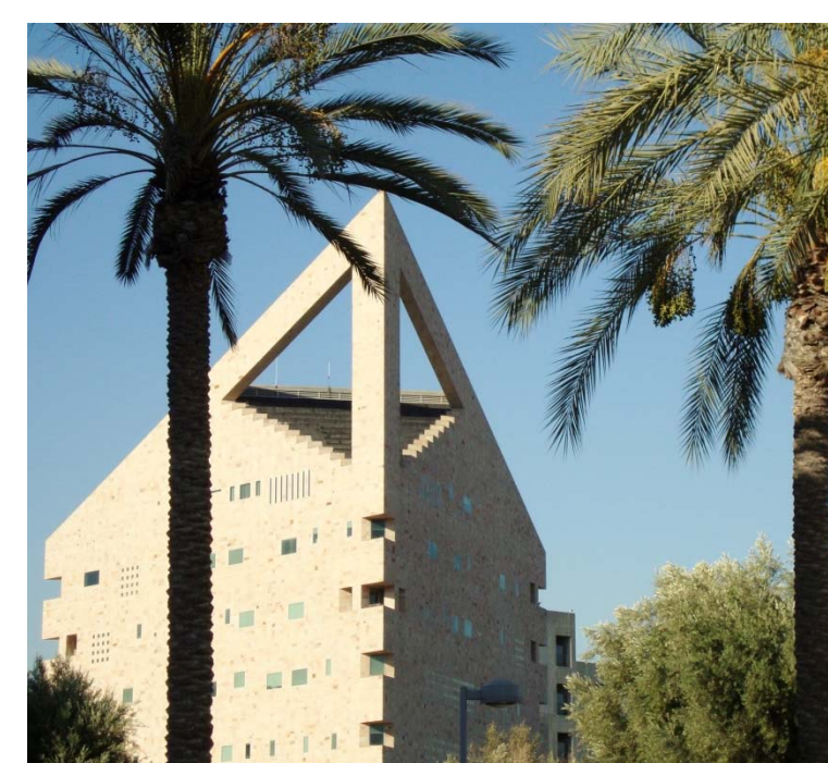
Figure 1. CPP CLA Building.
