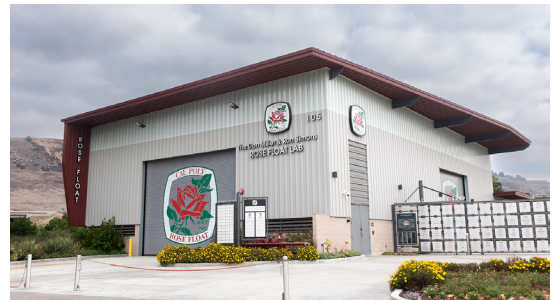
The Don E. Miller and Ron Simons Rose Float Lab and Design Complex opened at CPP in 2021 and provides 14,000 square feet of indoor and outdoor workspace.
