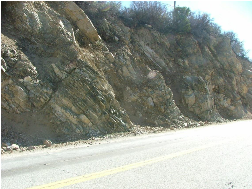
Figure 12. Photo of the New Mt Baldy Road cut facing southeast, within the felsic gneiss Megaclast
