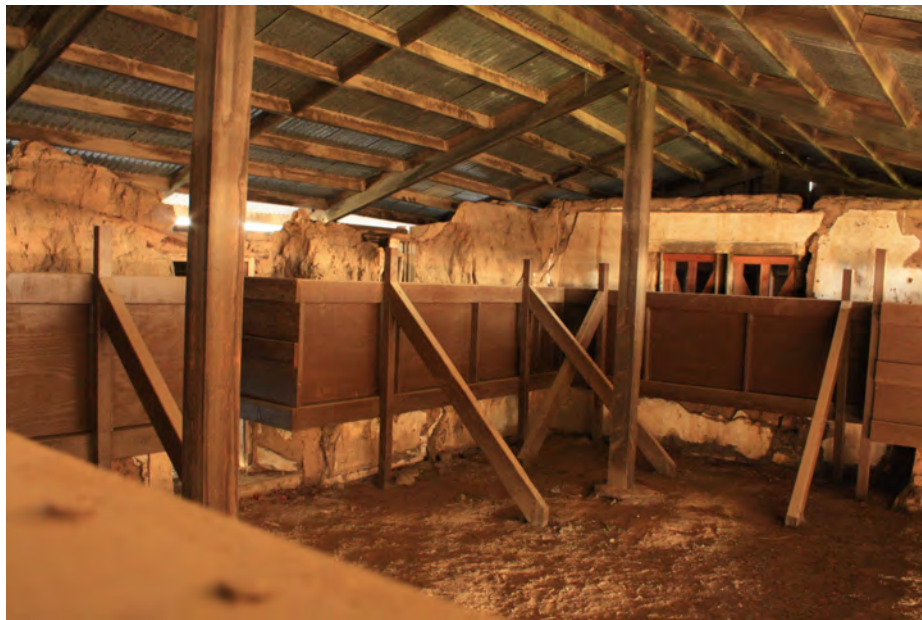
(a) All that remains of Trujillo Adobe. Walls are about 1-meter thick, composed of adobe bricks. Square shaped home, with approximately 10-meter long walls on each side.
