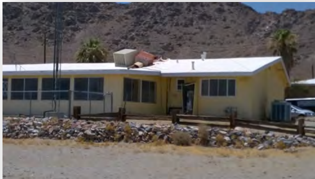
House damage after the Ridgecrest earthquakes, July 4th & 5th, 2019.
