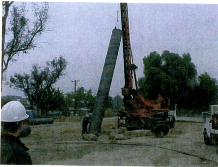
36-inch outside diameter steel conductor casing installation
