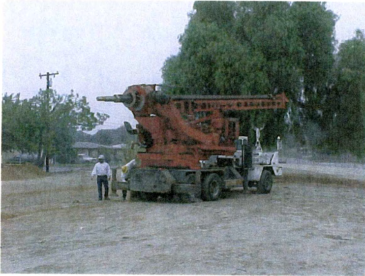
Bucket auger drill rig
