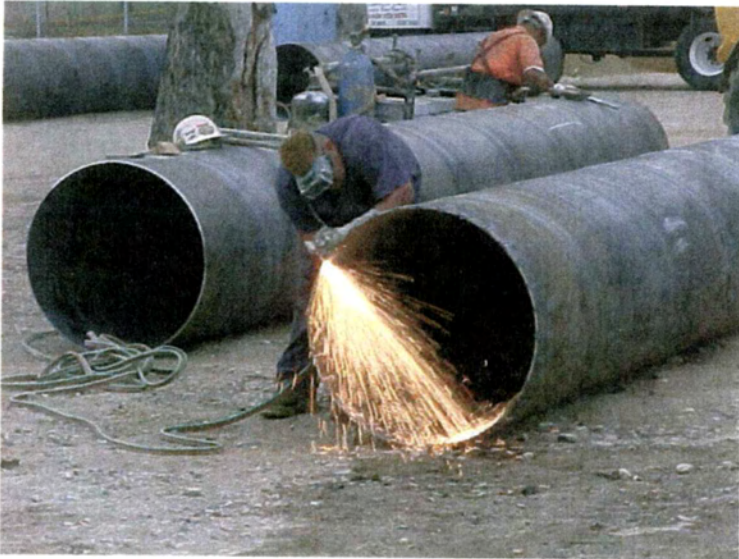
36-inch outside diameter steel conductor casing
