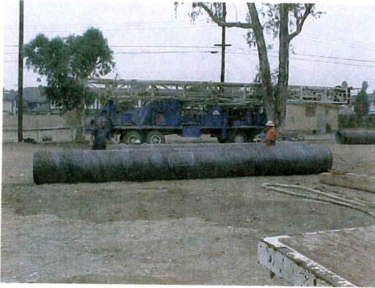
36-inch outside diameter steel conductor casing (50 foot section)
