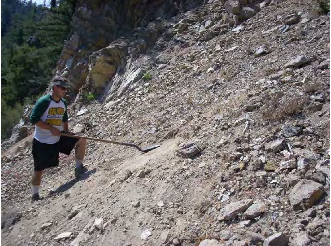
Figure 15. The basal slide plane is shown in the cleared section or slide and is roughly parallel to the shovel head.
