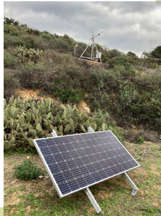
A solar panel powers the eddy covariance tower.
